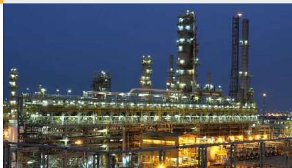
Laffan Refinery, Qatar
