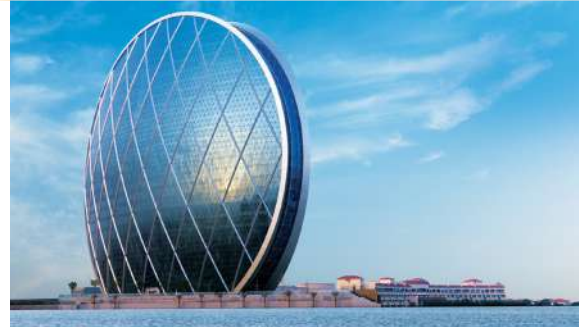
Aldar Headquarters, Abu Dhabi, UAE
