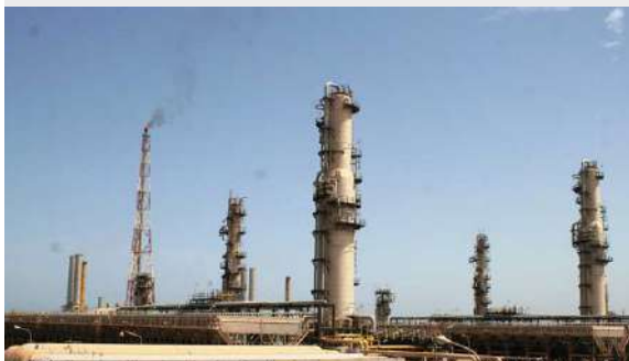
Sonatrach Petrochemical Plant, Algeria
